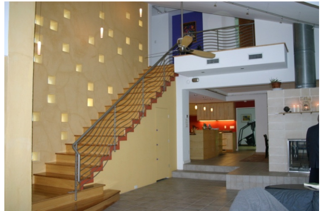
The windows on this staircase built by Ferrier Custom Builders in Fort Worth, Texas, let in natural light so less electric light is needed.
